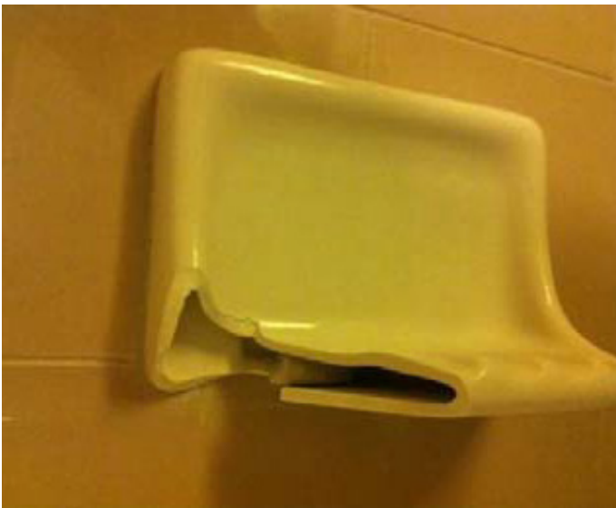
Chipped or broken soap dishes can pose a hazard
