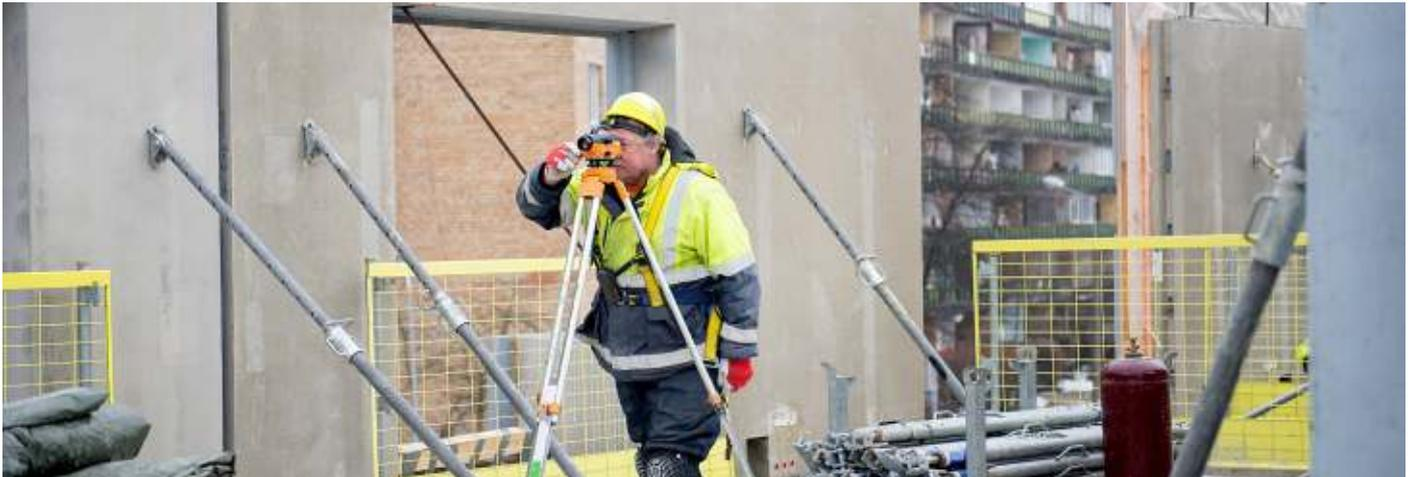
A site or contour survey is required prior to building to provide information on land levels, land contours, trees/vegetation and water and power services for accurate drafting of plans.
